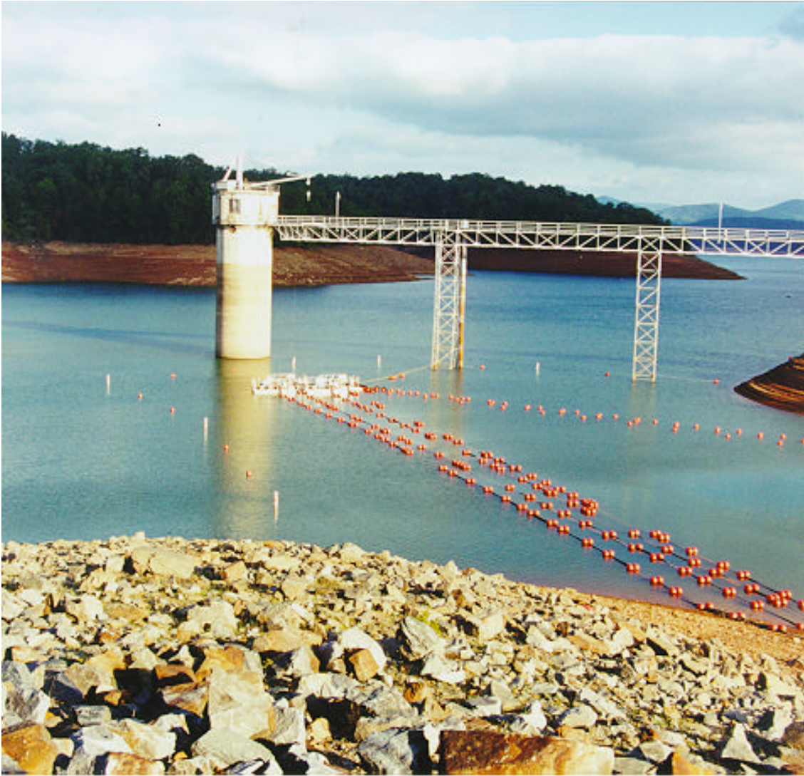
Blue Ridge Intake Tower Structure
